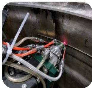
Bottom Ring On-Site Repair
