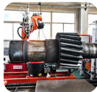
Transmission Shaft Repair
