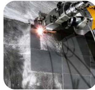
Runner Wear Plate Repair & Surface Reinforcement
