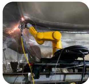
Runner Blade Surface Reinforcement
