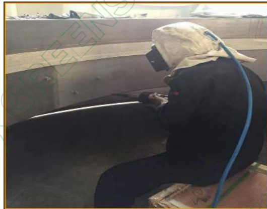
Shield center ring restoration size repair
